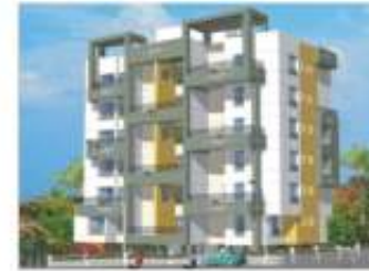
Welworth Celestina Near Station, Shivaji Nagar
